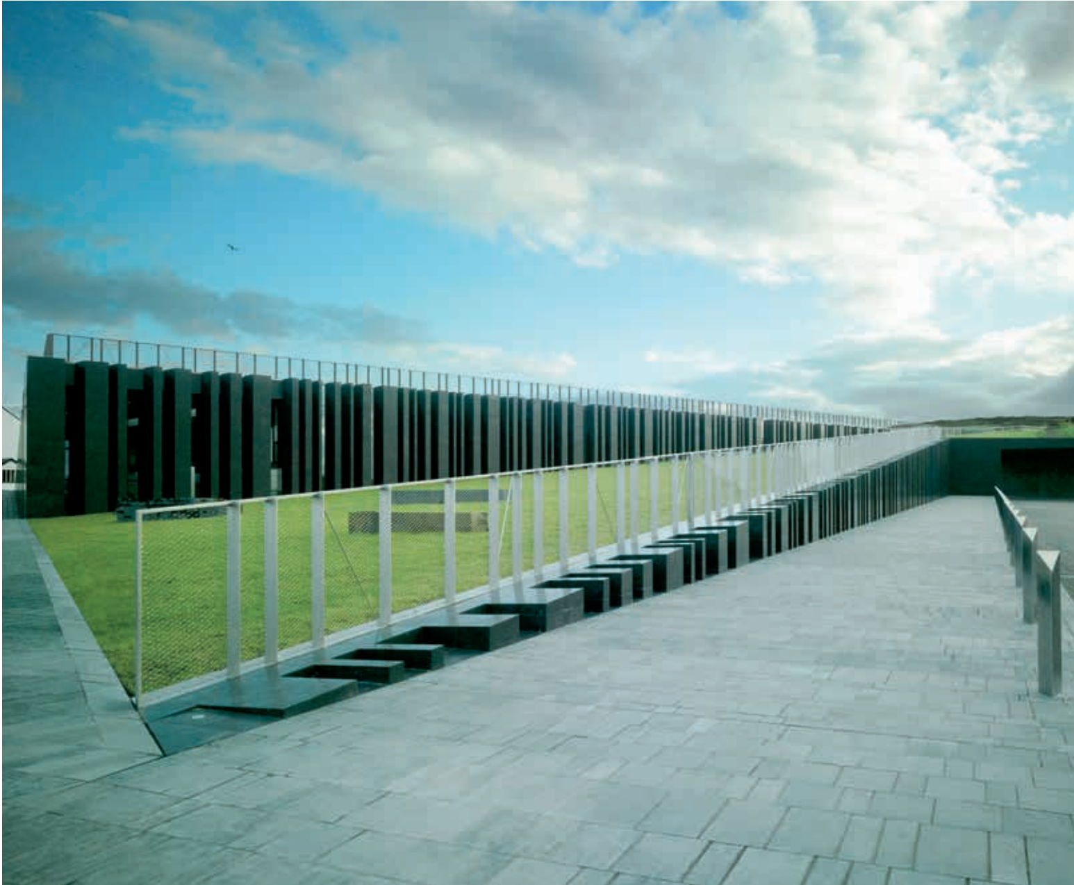
↑ The structure of the Giant's Causeway Visitor Centre comprises vertical stone mullions that echo the basalt columns which form the impressive coastal causeway and provide the inspiration for the area's name.
