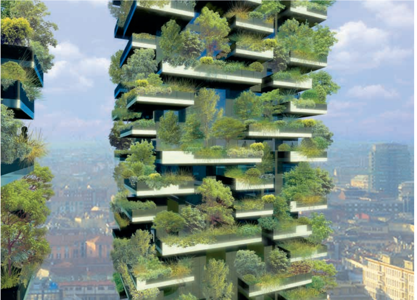
↑ The two “Bosco Verticale” residential towers will feature a living area of 50,000 square meters and 10,000 square meters of forest.
