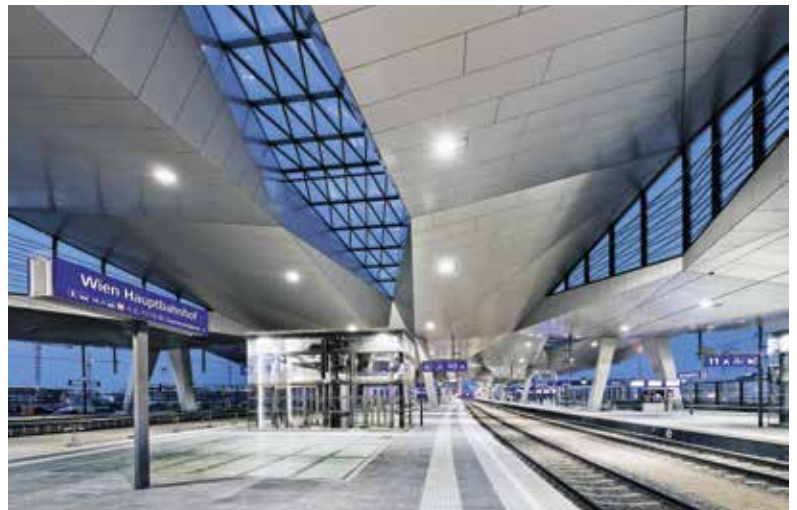
← Glass diamonds form skylights that provide lighting and ventilation.
