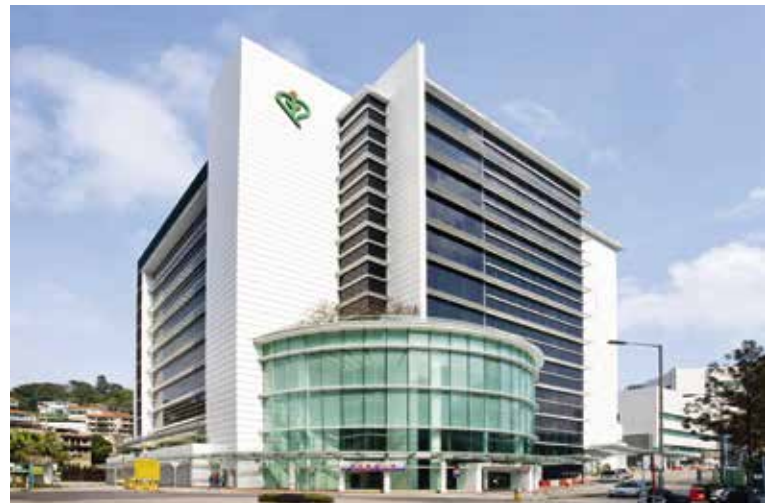
↑ The outpatient section of TKO Hospital ← Jepsen Building Products supplied a range of different products for North Lantau Hospital, including toilets, washbasins and urinals from Twyford.
