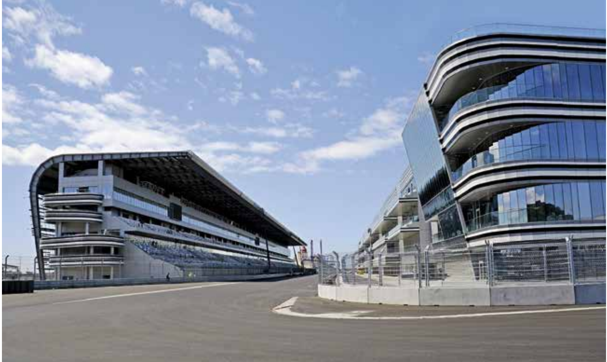
↑ A view of the grandstand and the racing circuit
