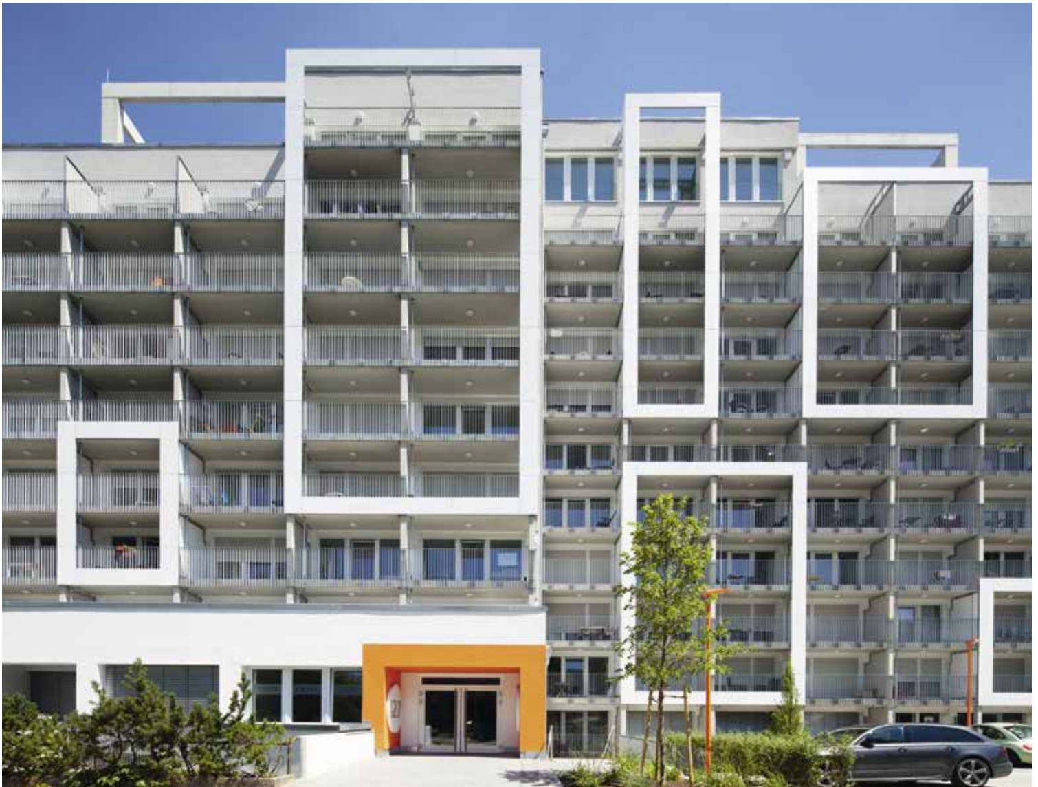
↑ Together with the balconies, the differently sized, geometrically arranged decorative beam structures represent an architectural highlight.
