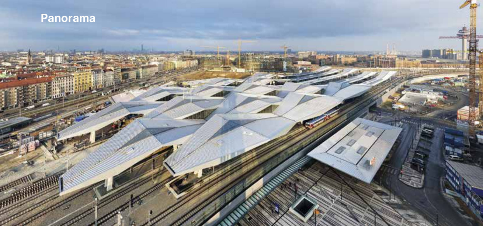
↑ A folded diamond-shaped roof extends over the platforms.
