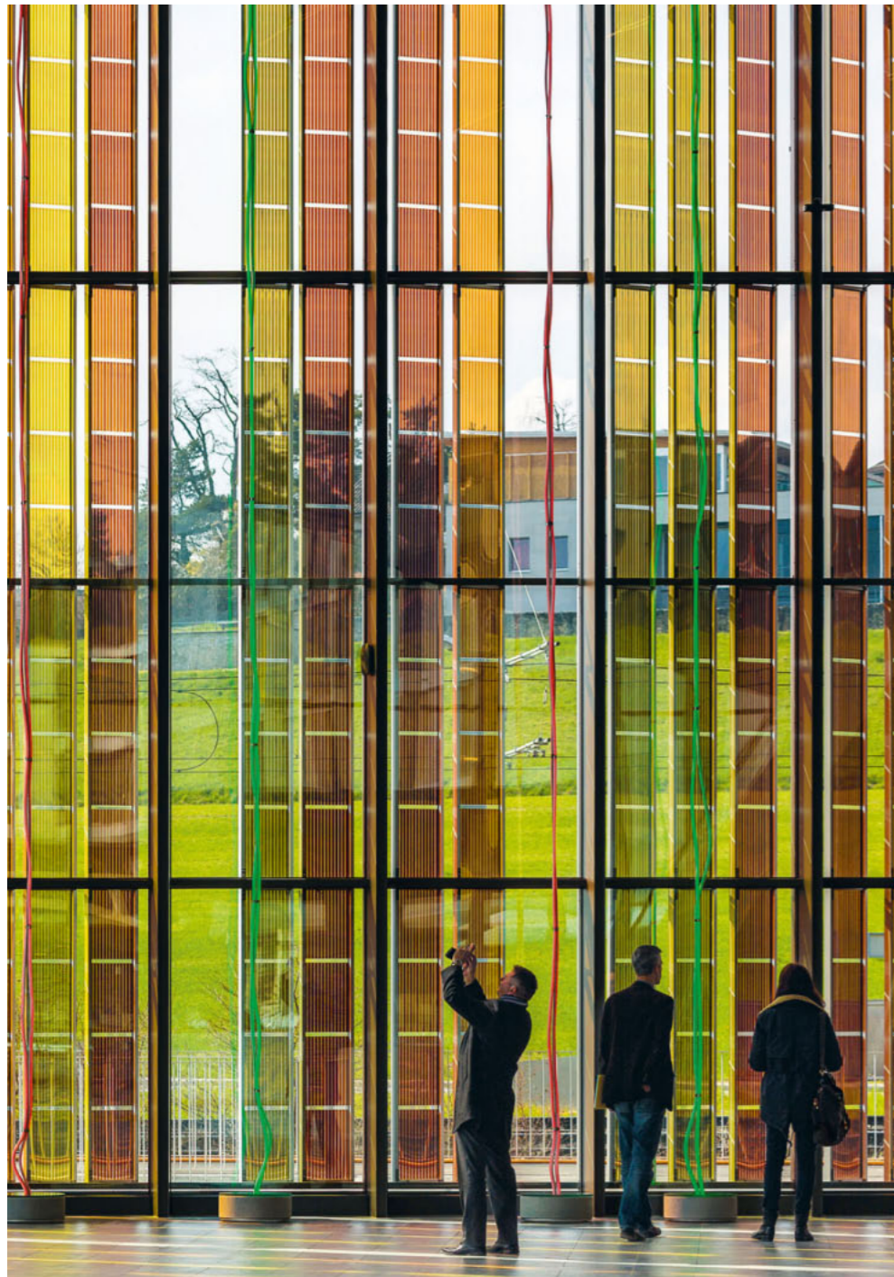
↑ The glass front of the new Convention Center features colorful solar cells that provide the green building with energy.
