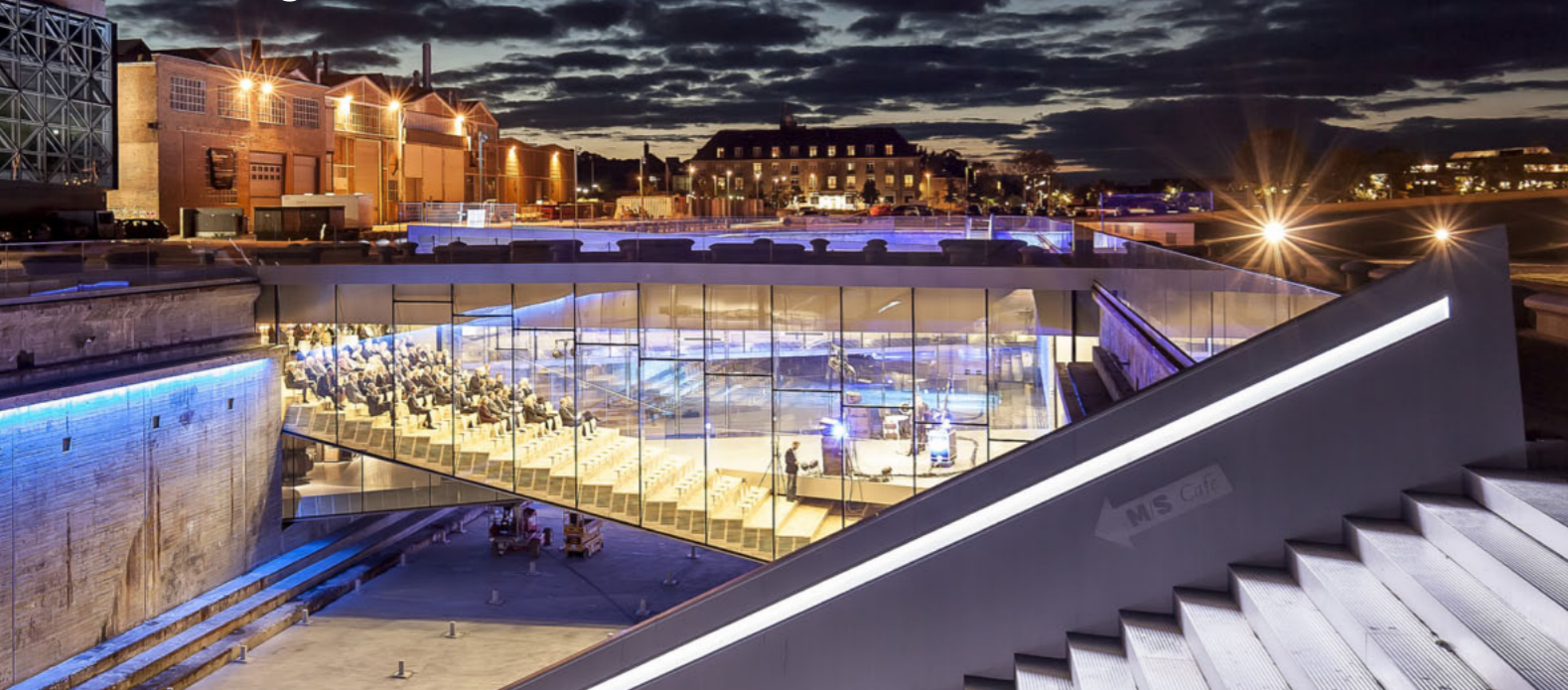
↑ As part of the museum construction process, the old dock wall was completely uncovered and the dry dock left empty.
