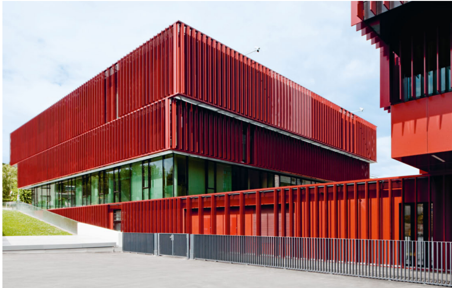
↑ The new building, which consists of two individual structures, features a striking dark red metal skin which also functions as outer bars.
