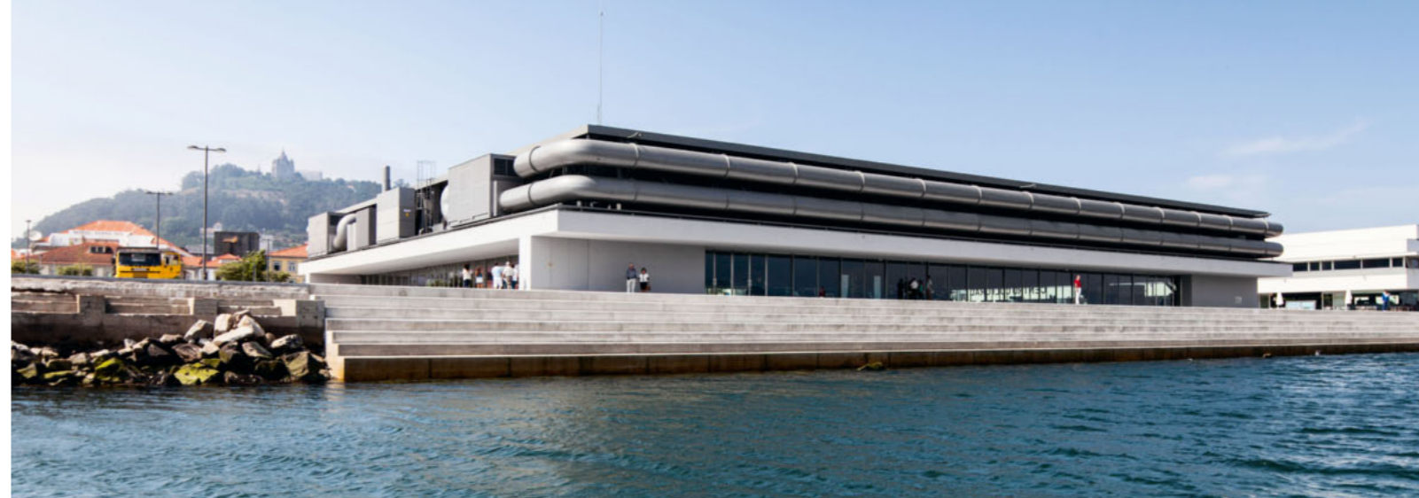
↑ Striking pipelines and metal superstructures on the roof, a multipurpose hall of sports and culture inside of it.
