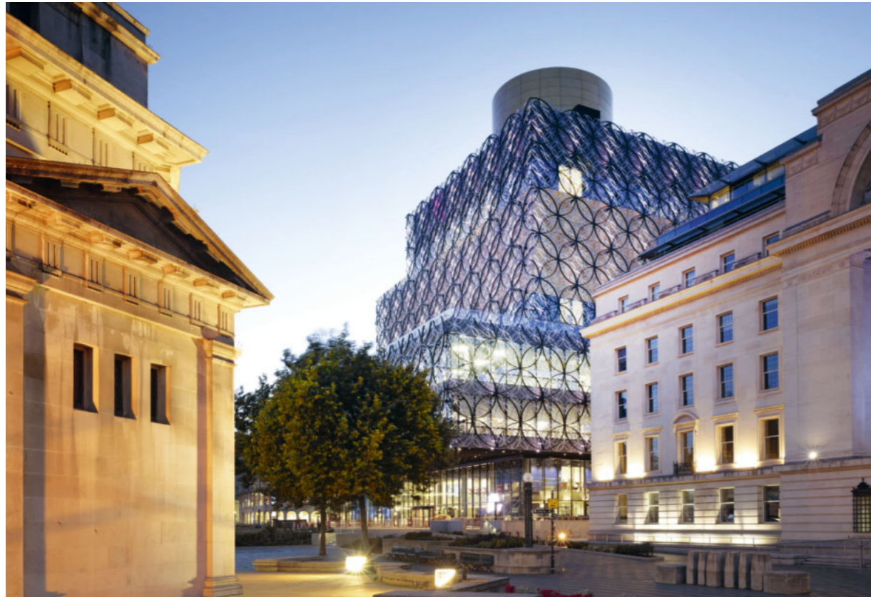
↑ The dominant structure blends into the urban context thanks to its striking ringed facade.
